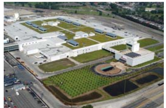
Ford's newly rebuilt Rouge Center in Dearborn, Michigan features a huge green roof.
